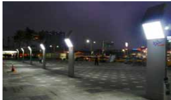
Street light at Guro Station
